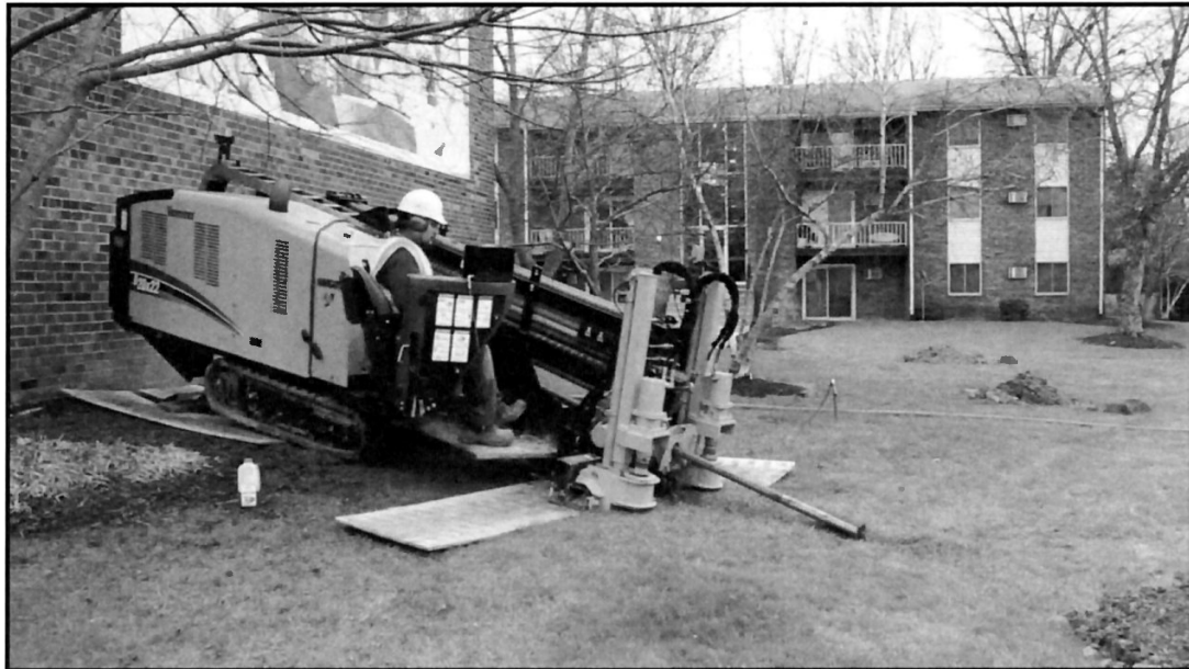
Plate 1-1: Typical Utility-Sized Horizontal Drilling Rig
