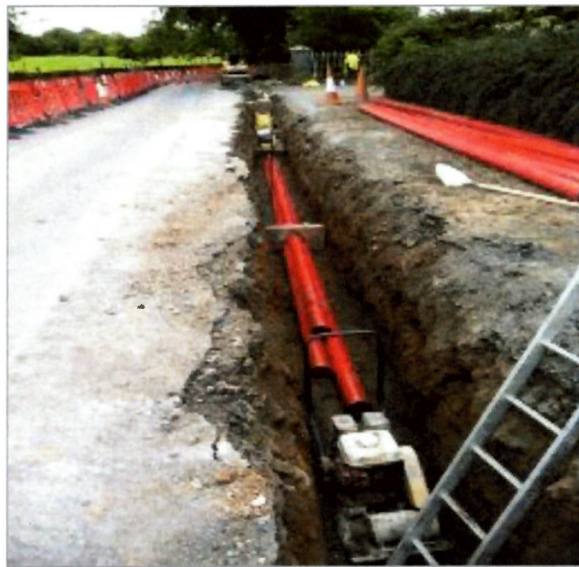
Figure 2 - Typical 110kV Underground Duct Installation
