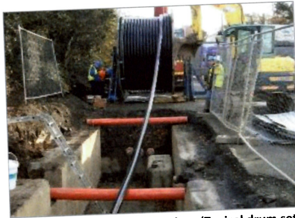
Figure 8 - HV cable pulling procedure (Typical drum set-up)
