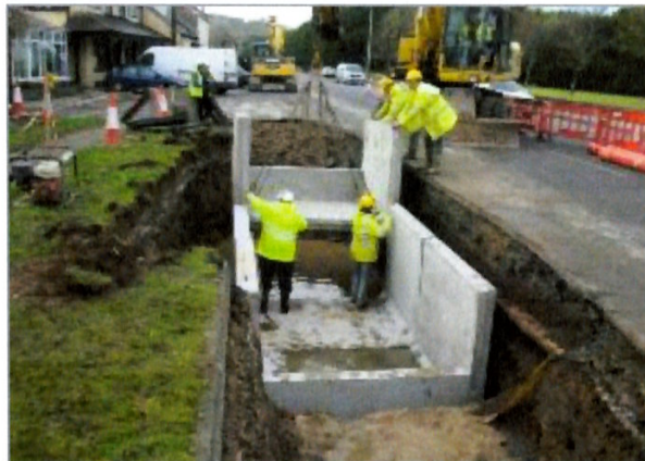
Figure 7 - Typical joint bay under construction (pre-cast)
